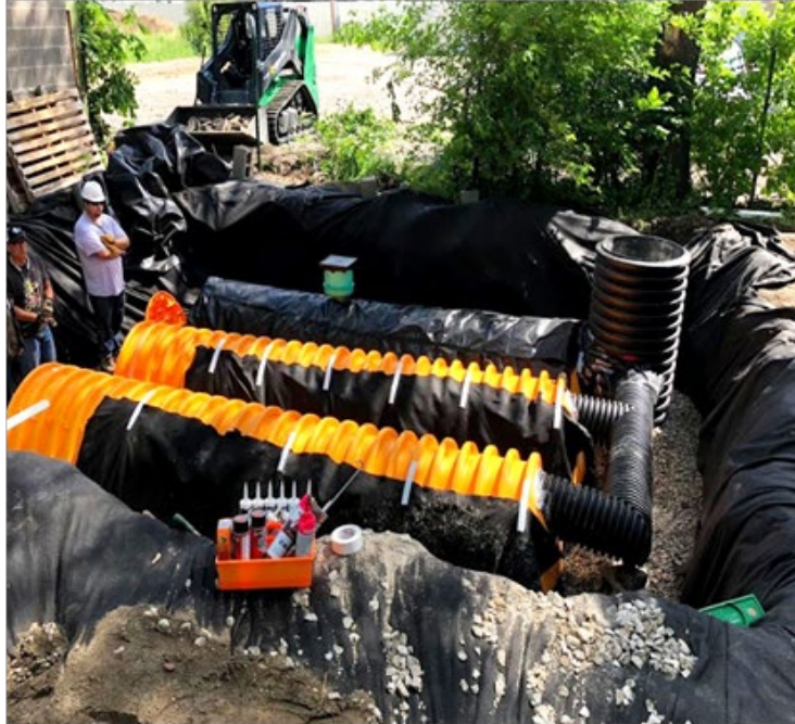
BELOW-GROUND CISTERN EXAMPLE
