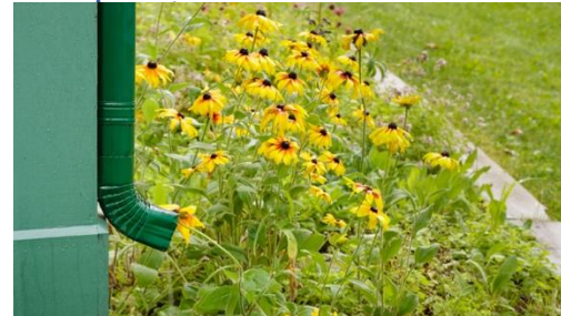
Disconnect downspout from sewer systems
